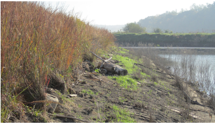
The roots of native prairie grasses protected the Mormon Bridge Embankment from erosion during the 2011 Missouri River flood; these photos were taken shortly after the floodwater receded. Photos courtesy of Dustin Ausdemore.
