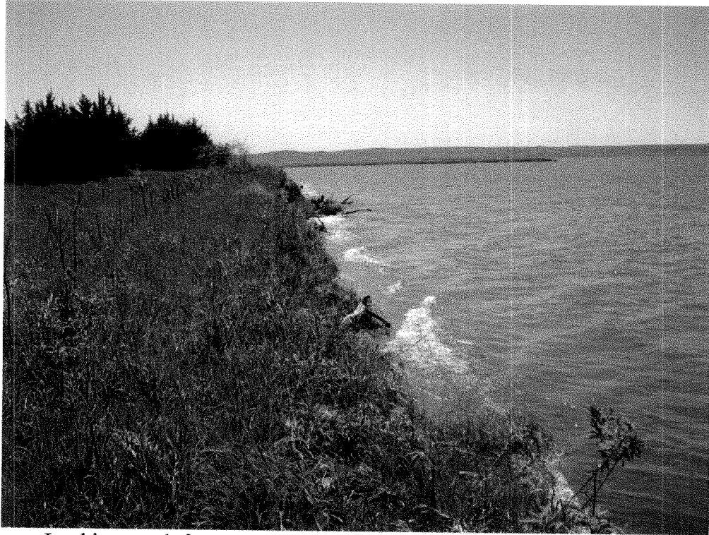
Looking south from area where northern part of dike will be located.
